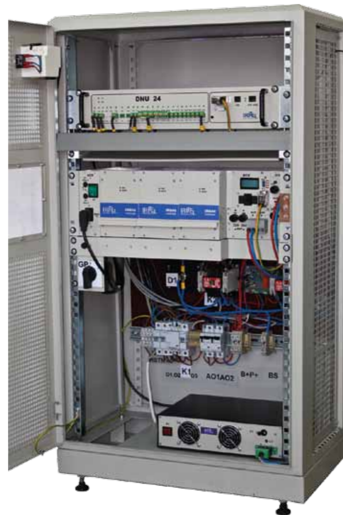
SN12/110 with extra battery charging, additional devices and system for remote monitoring and control (DNU24) in one cabinet (1000 mm)
